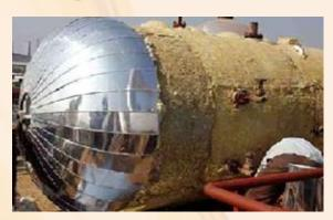
All insulation shall be done by ROCKWOOL mattress50mm thick as required of Density 100Kg/cu mtr of reputed make and cladded with aluminium / GI sheet 24 gauge. This part of the job shall be done on the site. The material shall be supplied loose and client has to organize the same at site under our guidance. Insulation of pipelines below blenders to filling lines to be done on site.
